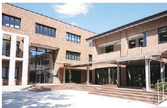
IMO棟1及び2 IMO Building 1 and 2
